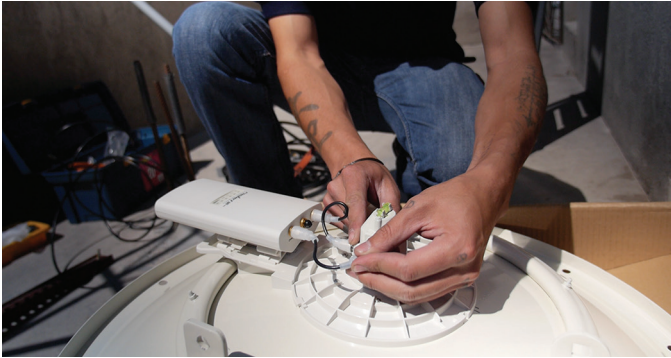
Connecting the RF cables from the RocketM to the RocketDish
