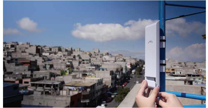
Installing a NanoStationM
